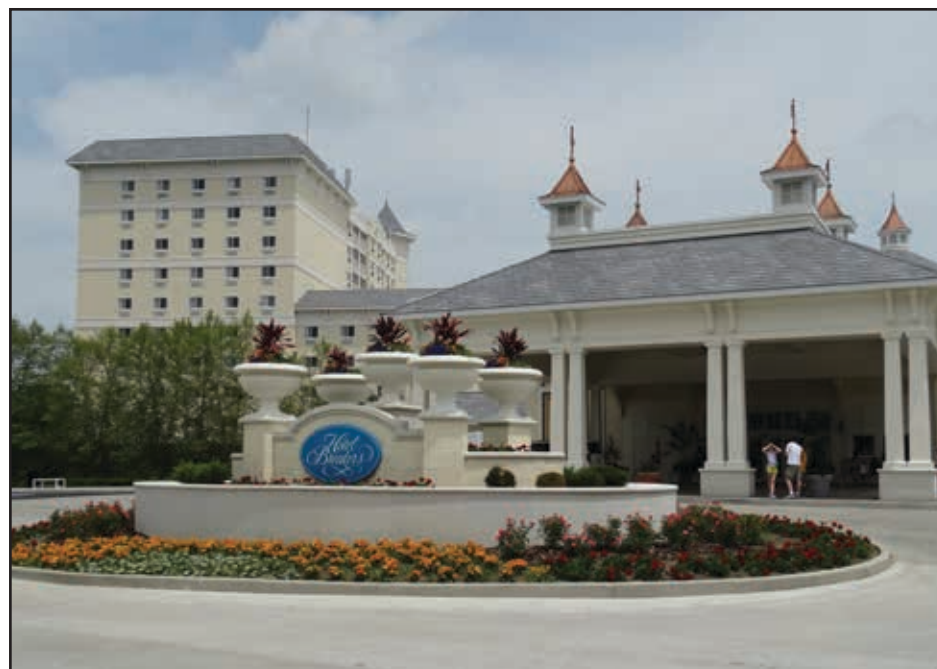
Cedar Point has seen more than $180 million in improvements at the resort property over the last five years. Among the upgrades enjoyed by vacationing guests are the complete makeover and rebuild of the historic Hotel Breakers, shown here. AT/ TIM BALDWIN
