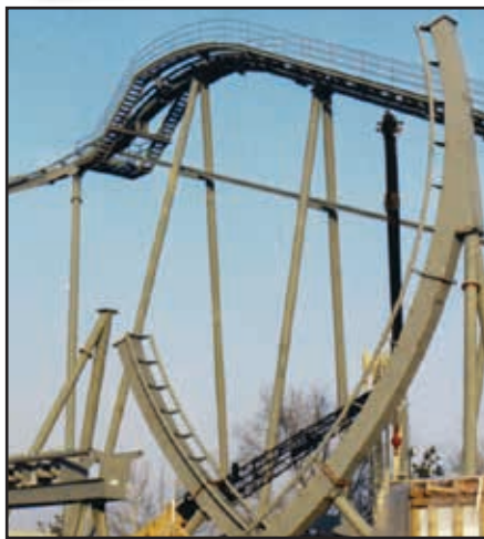
B&M's first full coaster project was Iron Wolf, shown here under construction in 1990 at Six Flags Great America. AT FILE
